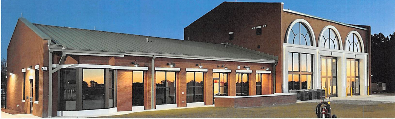
Coastal Carolina Regional Airport in New Bern opened a $5.8 million aircraft rescue and firefighting facility in 2021.
